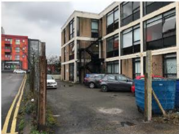
4 | View looking north-west from rear of site
