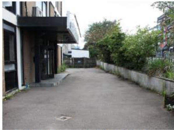
2 | View looking south-west towards existing building main entrance
